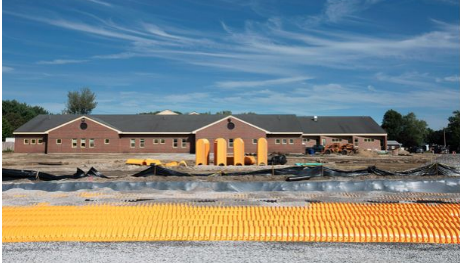
A drainage system for a future athletic field at Saccharappa Elementary School is just a small part of the renovation project. Staff photo by Ben McCanna
